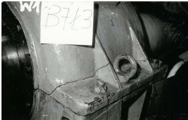
Fig. 1. A crack in upper casing of shaftline bearing
