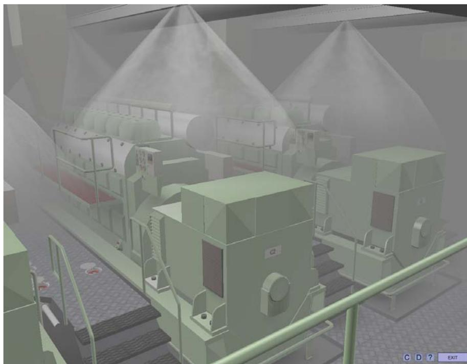
*Fig. 10 Water mist activation in Diesel generators section*
